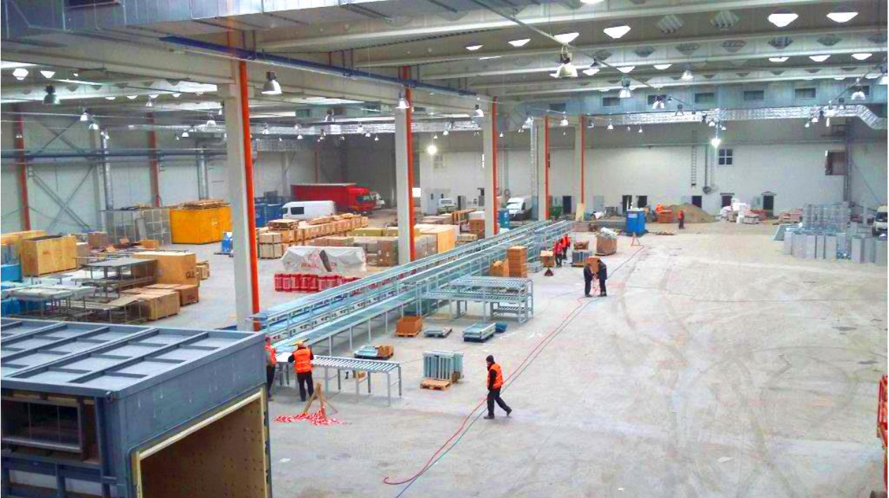
Progress at Plant 4 in Stalowa Wola, Poland
